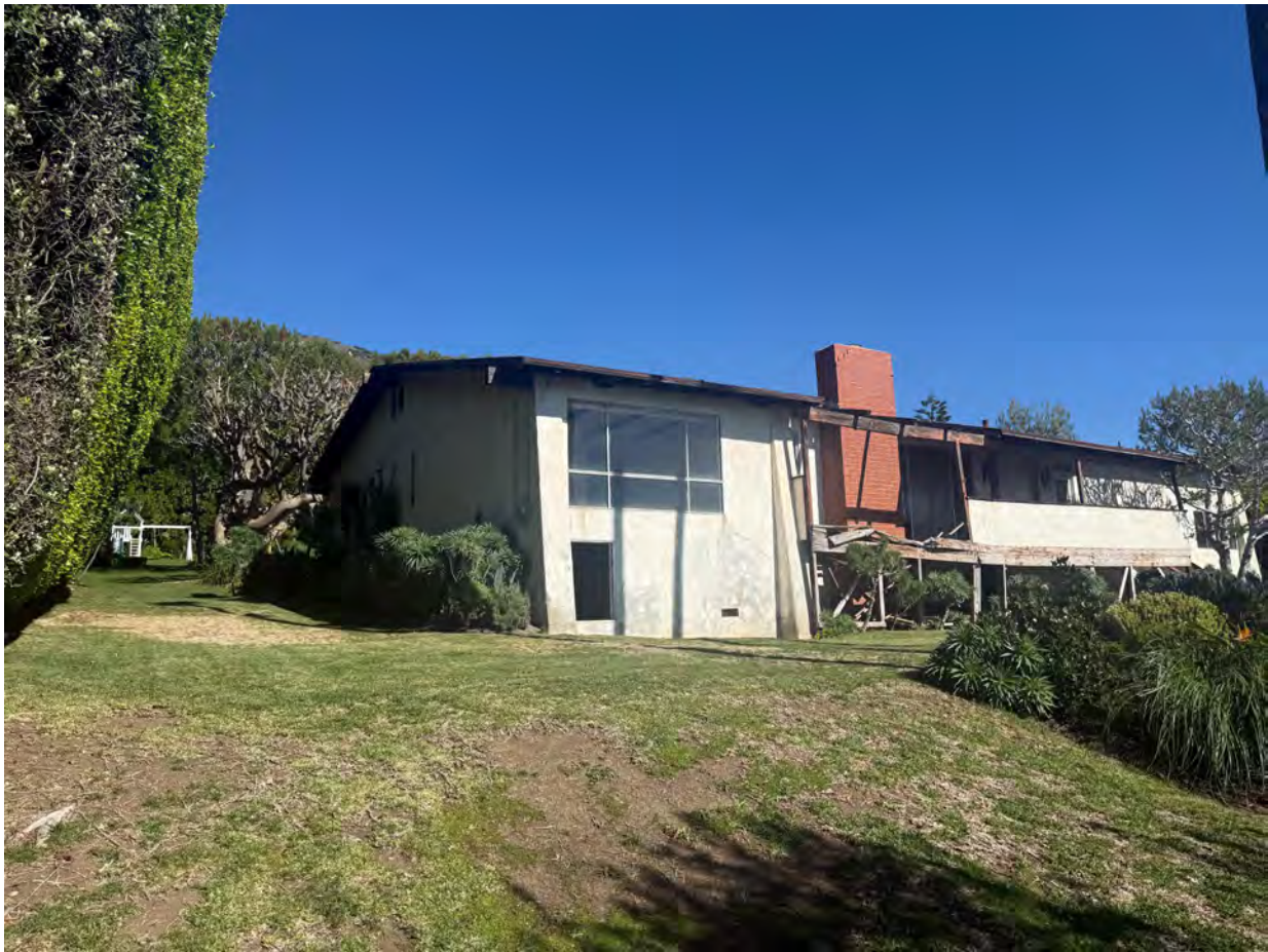
View looking northeast Existing SFR
